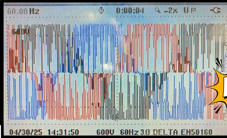
6-pulse VFD PWM voltage output
